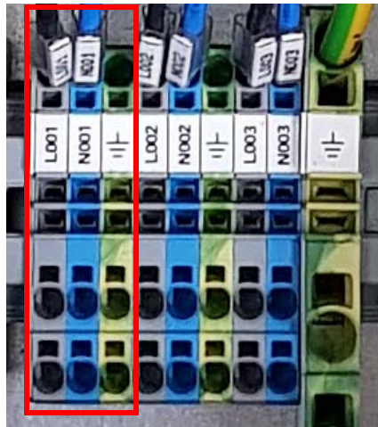
Figure 5 - Terminal Block for Out#1 and Out#2
