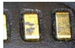
Damaged contacts on other devices
